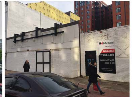
EXISTING BRICK FACADE
