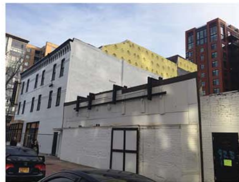
EXISTING BRICK FACADE
